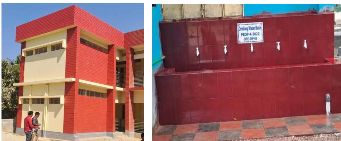
Fig. 10 (L): Constructed Wash Block (R): 5 outlet water collection basin
